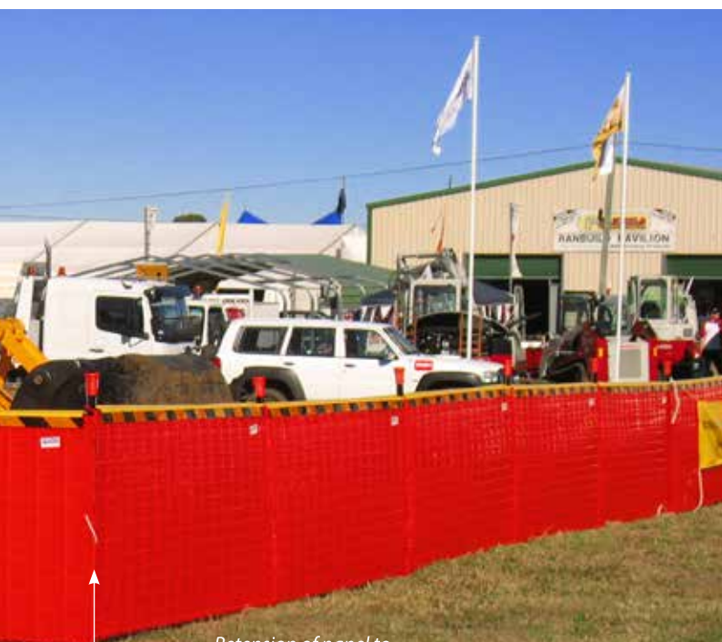
Retention of panel to star picket with cable tie
